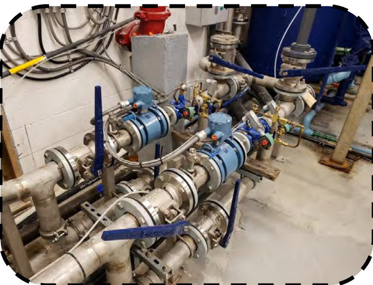
Meegwetch, Allan Dupuis Water Plant Operator Public Works Manager
