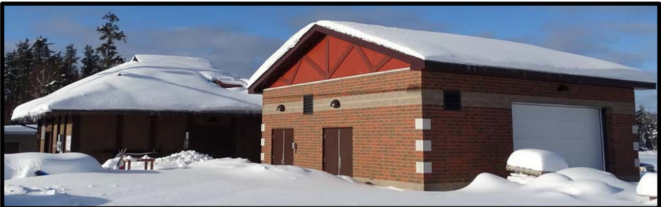
Water Treatment Plant Upgrade Progress
